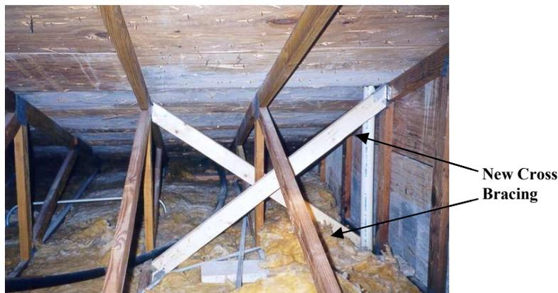
**Figure A-10. Gable End Bracing Secured with Metal Connections.**
