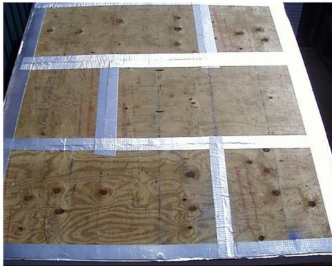
**Figure A-3. Self-Adhering Modified Bitumen Strips Applied to Plywood Joints of Roof Deck**
