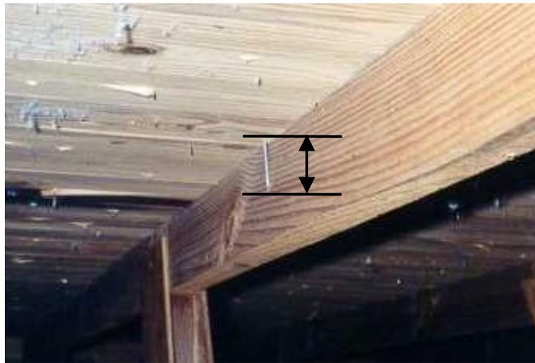
**Figure A-7. Roof Deck Attachment Rating Requires an Attic Inspection.**
