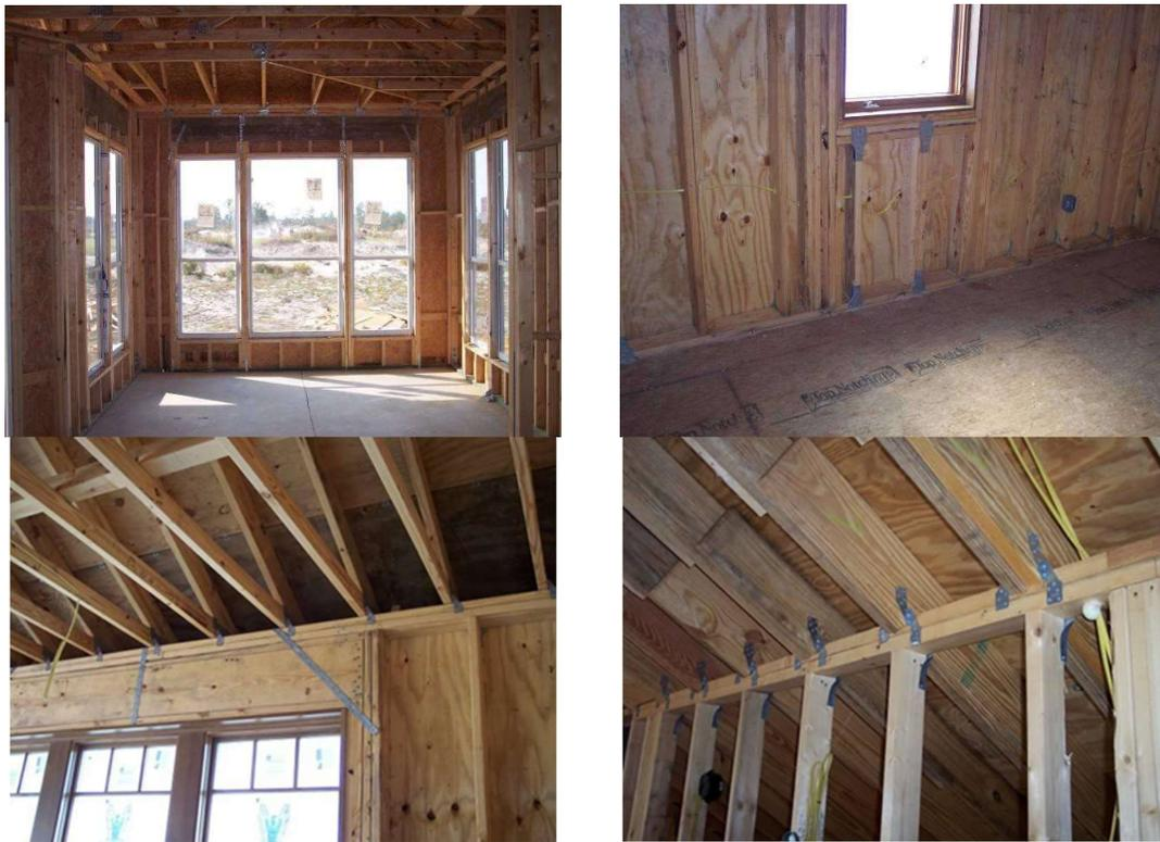
**Figure 2-41. Framing and Connection Details for FBC Gable Roof Home.**
